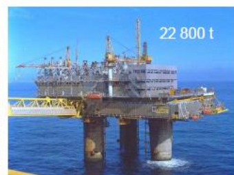
TCP2 Production Platform
