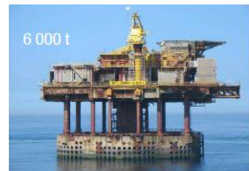
CDP1 Drilling Platform
