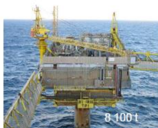
TP1 Production Platform
