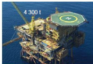
DP2 Drilling Platform
